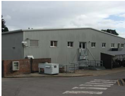
CE building (B57)
