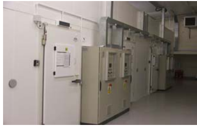
Containment rooms B63
